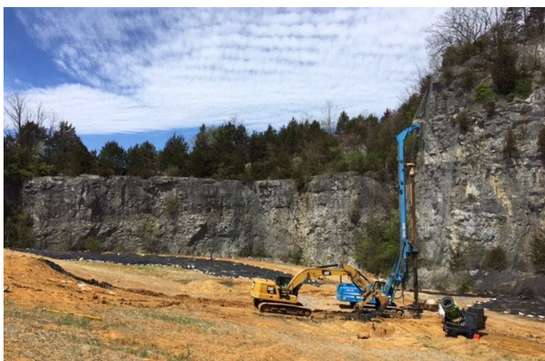
Drilling EW-70, installed SOMS liner in the background
