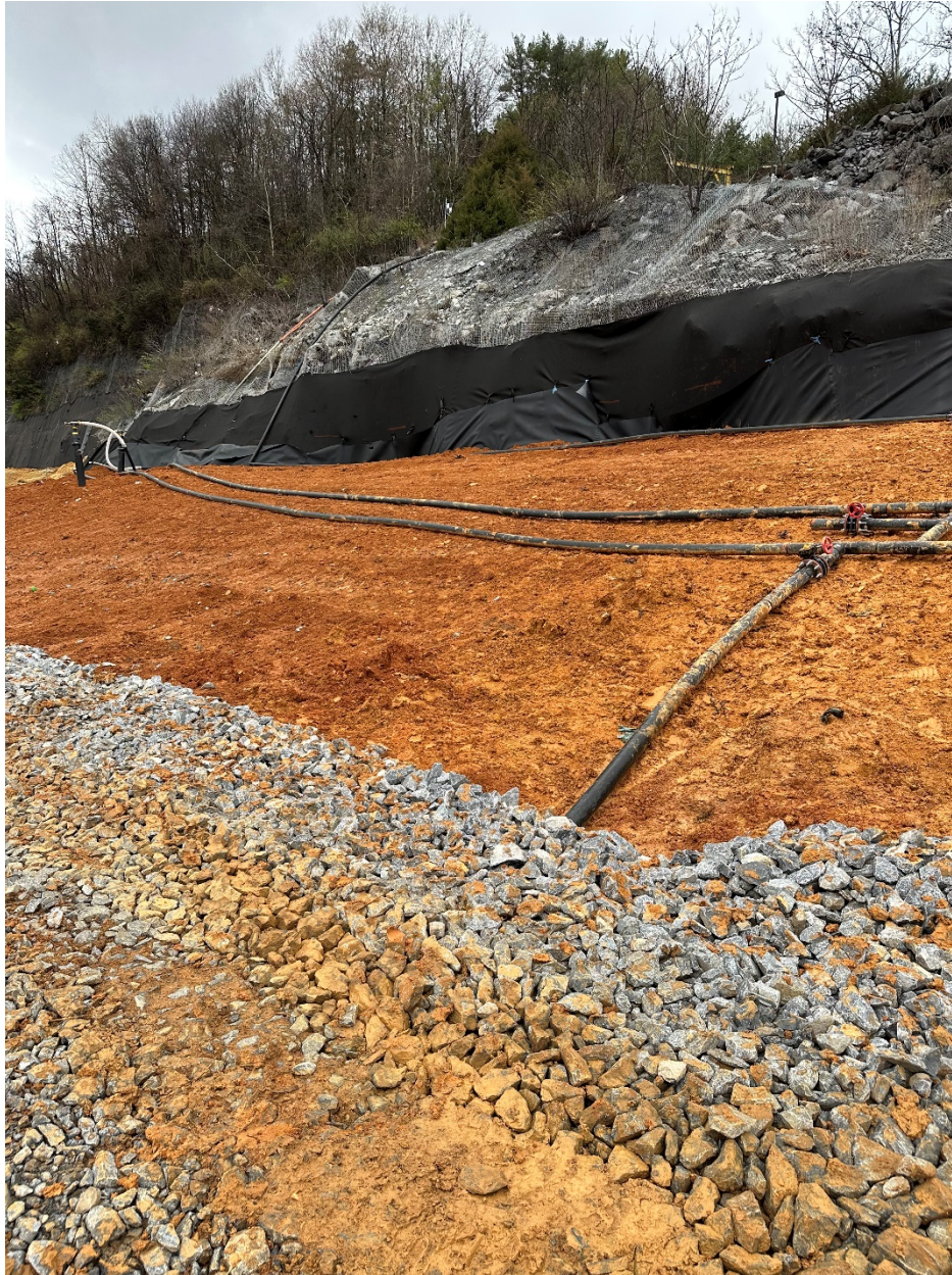
Figure 8. Phase 1 Sidewall Odor Mitigation System Construction
