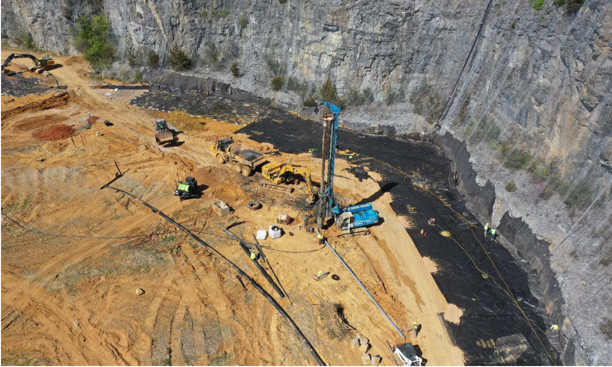
Figure 5. Landfill Gas Extraction Well Drilling
