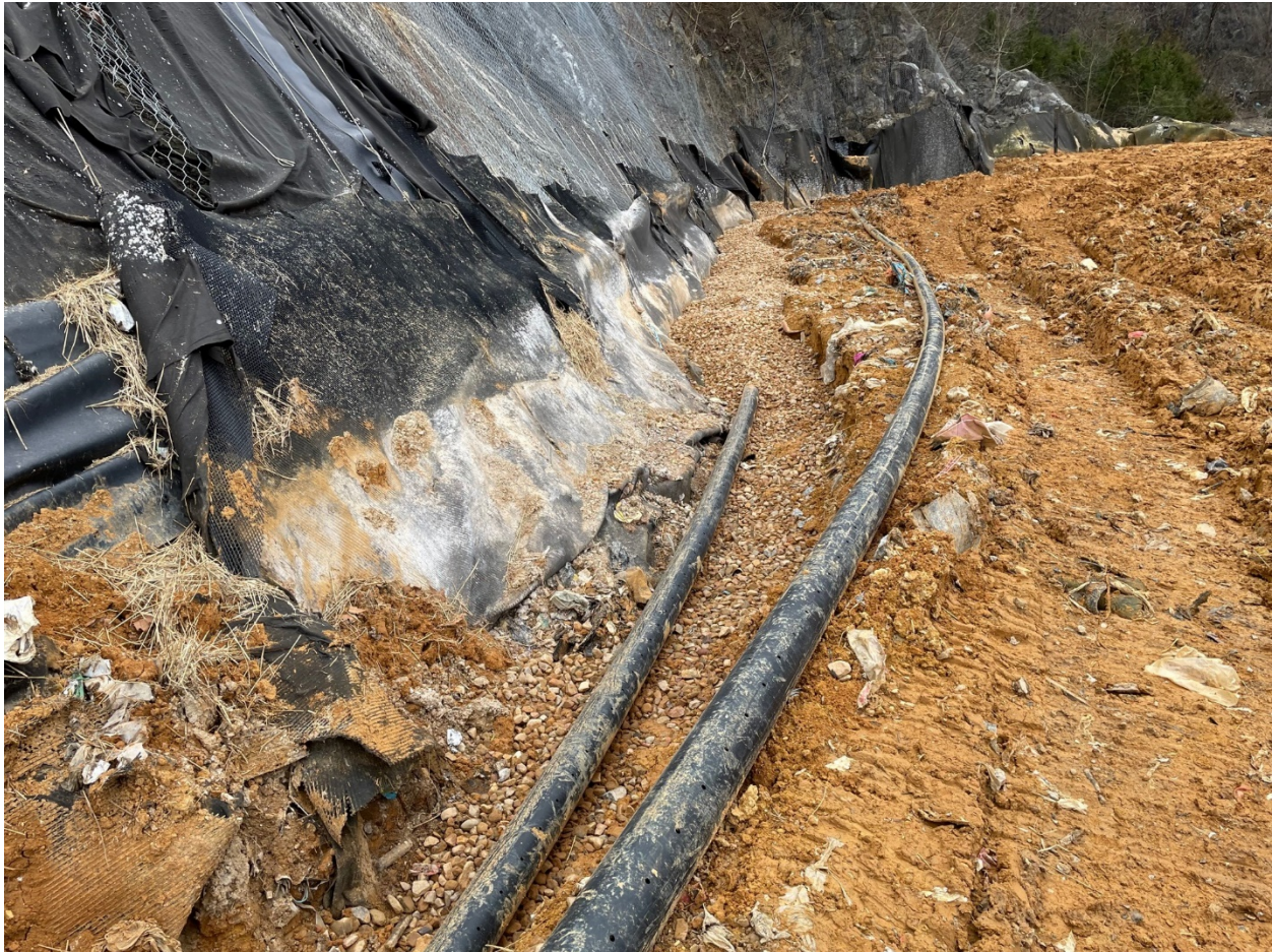
Figure 2. Phase 2 Sidewall Odor Mitigation System Construction
