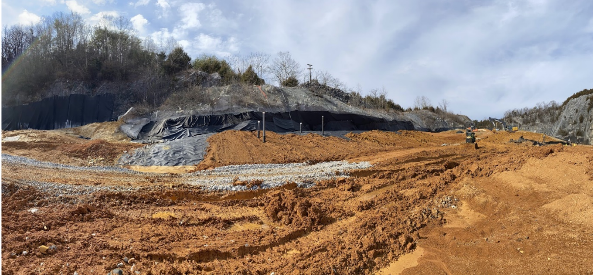
Figure 1. Phase 1 Sidewall Odor Mitigation System Construction
