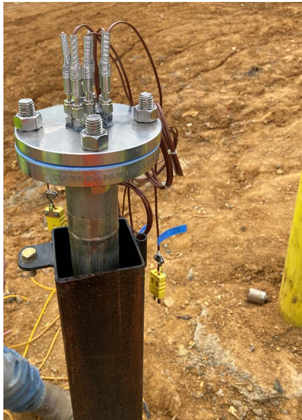
Figure 3. In-waste Temperature Sensor Installation
