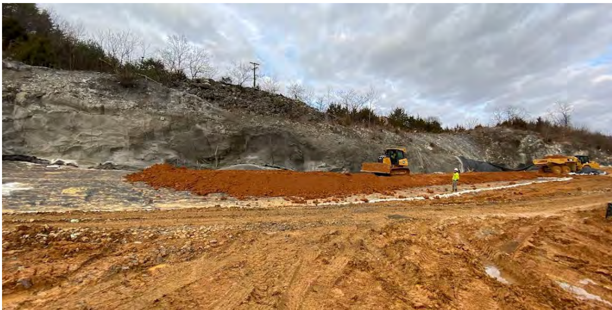
Figure 1. Sidewall Odor Mitigation System Construction
