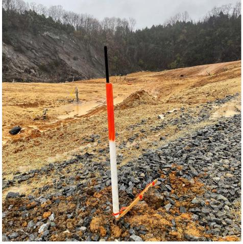
Figure 3. Settlement Plate after Installation
