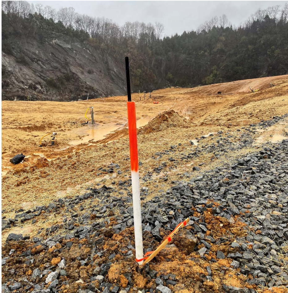
Figure 12. Settlement Plate after Installation
